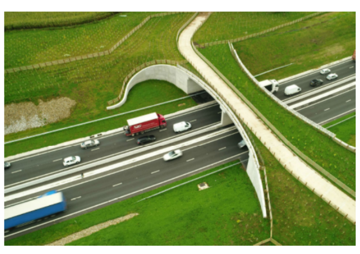
Potential to provide green bridge by widening deck and incorporating vegetation. Consideration would need to be taken regarding drainage and the increased load on the bridge.
